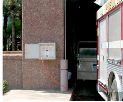
Figure 12.7. An exterior FDCP being supplied by a fire service mobile air unit.
