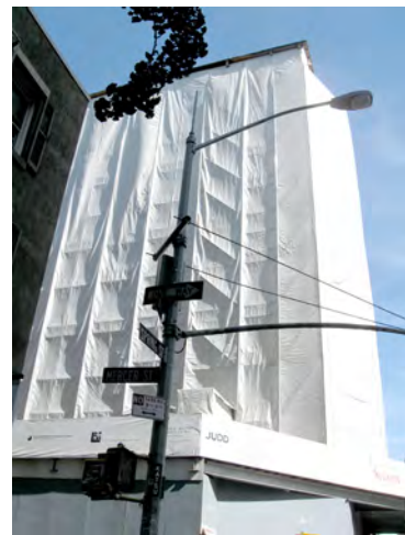
Figure 13.16. A temporary barrier covering an entire building.
