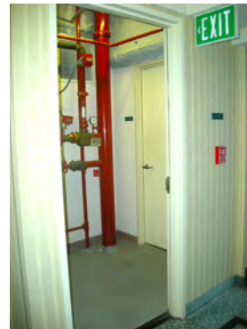
Figure 9.17. A standpipe riser and a FHC in a vestibule. The corridor door (foreground) can remain open for hose line use while the stair door (background) remains closed.
