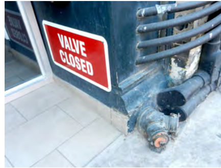
Figure 13.15. A sign next to an FDC indicating that the system valve is shut off.
