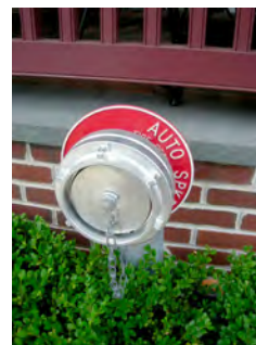
Figure 10.5. A quick-connect type of FDC.
