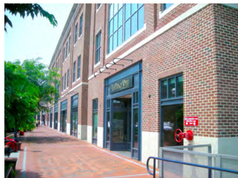
Figure 9.12. A pedestrian promenade serving ground-floor tenant spaces with no fire apparatus access. Below the red control valve is an exterior FHC.
