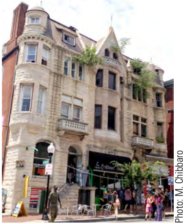
Figure 13.17. A building deteriorated to the point that trees are growing in it and major cracks are apparent.
