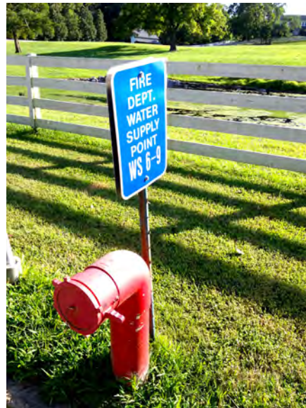
Figure 4.2. A dry fire hydrant piped to the lake in the background.
