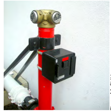
Figure 10.6. An FDC with locked plugs. The key is in the key box below the inlets.
