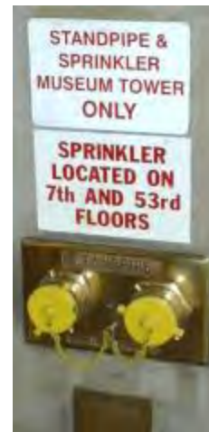
Figure 10.16. An FDC sign showing partial system coverage.
