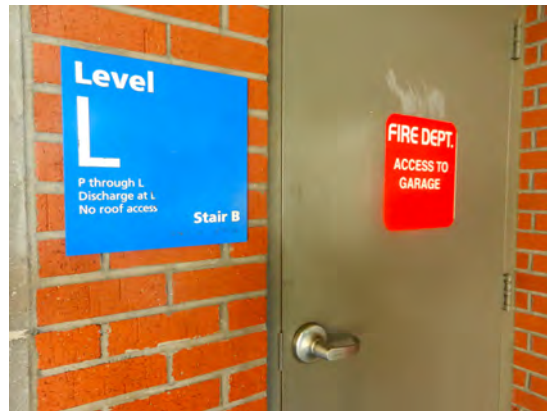
Figure 6.10. Signs outside a stair discharge door indicating fire service access (right) and the levels served by the stair (left).
