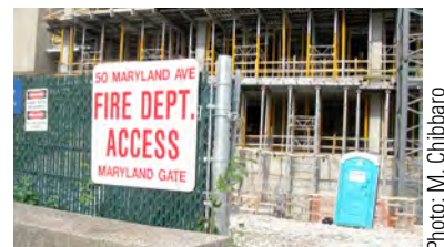
Figure 13.5. Temporary fire apparatus access.
