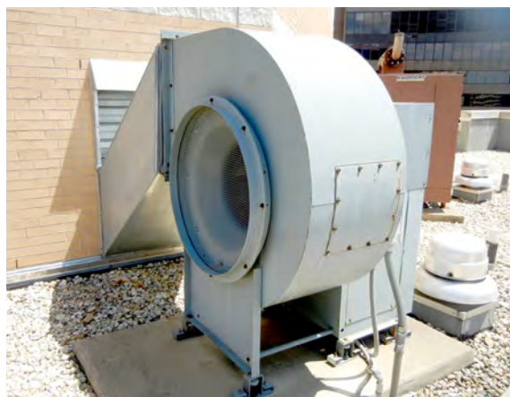
Figure 12.12. A stair pressurization fan.
