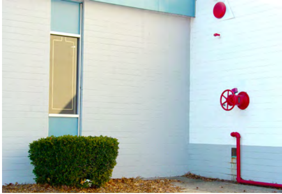
Figure 8.5. A wall control valve next to a window. Fire issuing from this window could prevent access to the valve.
