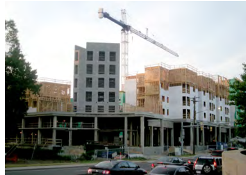
Figure 13.4. Firefighters can obtain valuable insight about construction materials and methods as a building is being built.
