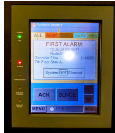
Figure 11.3 A textual-style annunciator panel with a touch-screen display.
