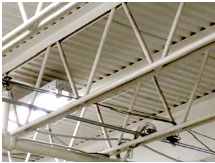
Figure 7.6. Steel bar joists.
