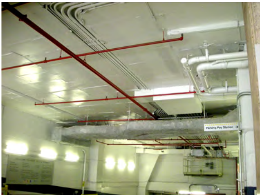
Figure 8.1. A fire sprinkler system.
