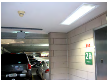
Figure 11.9. A smoke detector mounted in an outdoor location (an open parking garage).
