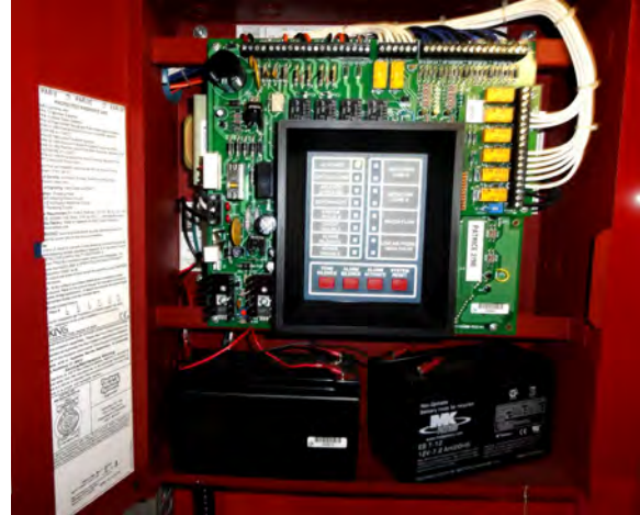
Figure 11.1. A basic fire alarm control panel with its door open, showing the wiring and the batteries for backup power. The controls and indicator lights in the center are visible when the panel door is closed and locked.
