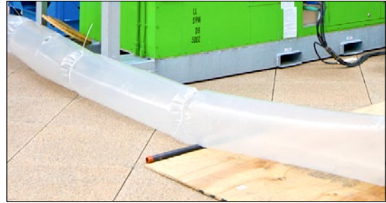
Lay-flat ducting in use
