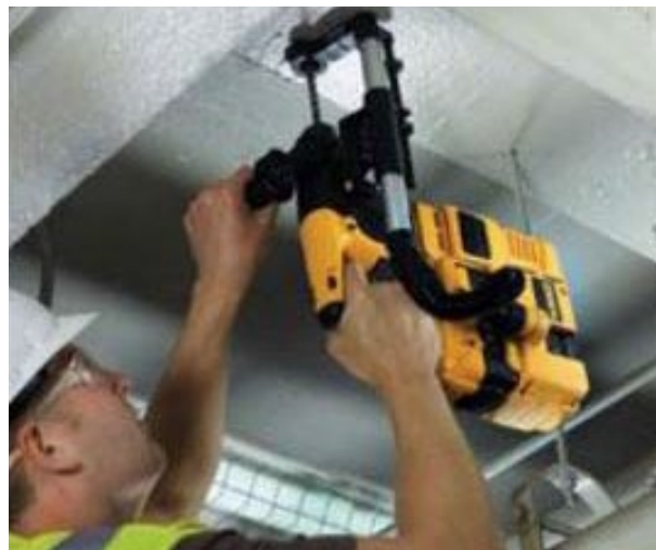
Worker drilling into concrete with a rotary hammer equipped with shroud and dust collection system. Note the shroud around drill bit, silver and black hose, and dust collector are attached conveniently to the drill.
