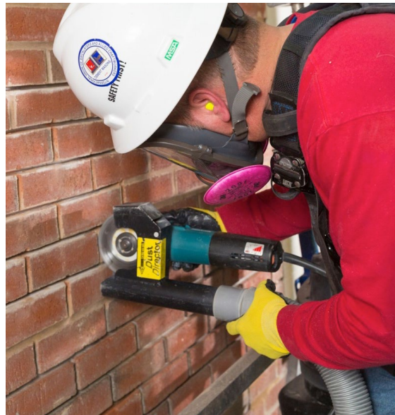
Worker grinding mortar from between bricks with a handheld grinder equipped with a shroud and dust collection system. In addition, worker is using respiratory protection.
