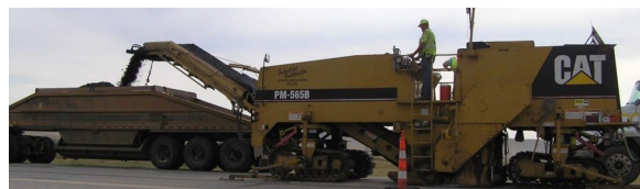
Milling machine milling asphalt road and loading debris into a haul truck. Photo courtesy of NIOSH. The equipment shown in this picture is for illustrative purposes only and is not intended as an endorsement by OSHA of this company, its products or services.
