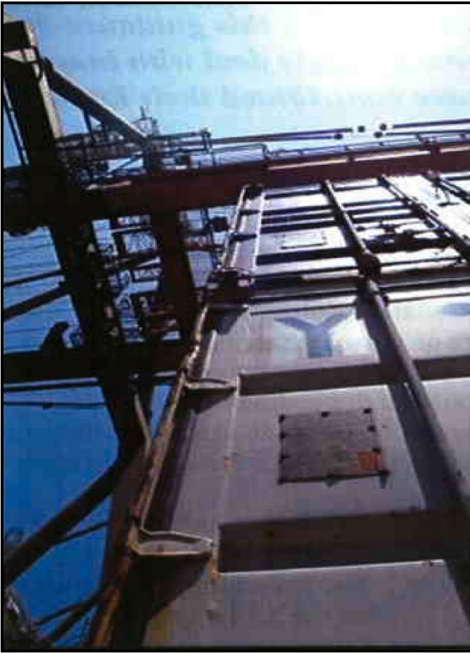
Foreman must direct the crane operator's movement.
