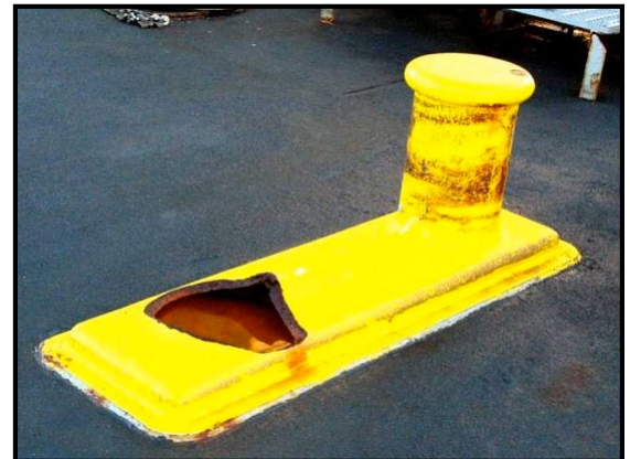
Figure 1. A hollow area under a mooring bitt.
