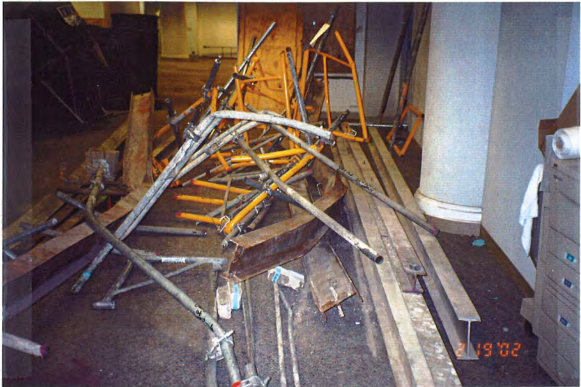
Figure 3-27. Condition of the Recovered Scaffold Frames, Lateral Bracings, and Bottom Support Members I.
