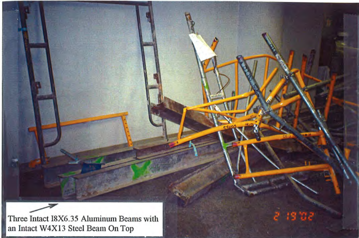
Figure 3-29. Condition of the Recovered Scaffold Frames, Lateral Bracings, and Bottom Support Members III.
