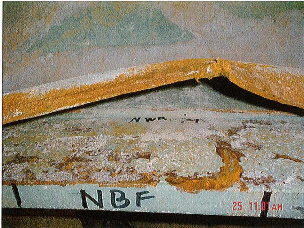
FIGURE 34 (North girder bottom flange)
