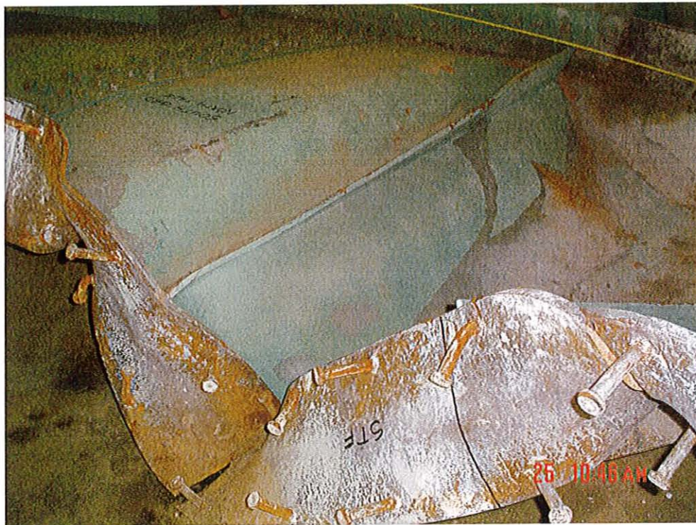
FIGURE 31 (south girder top flange)
