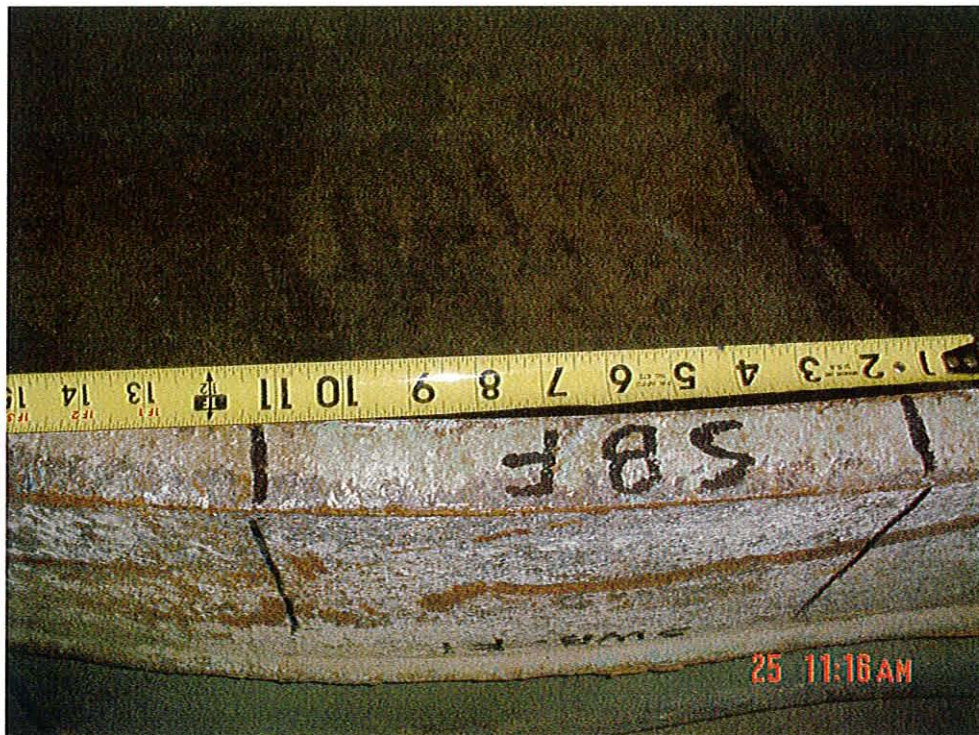
FIGURE 35 (South girder bottom flange)
