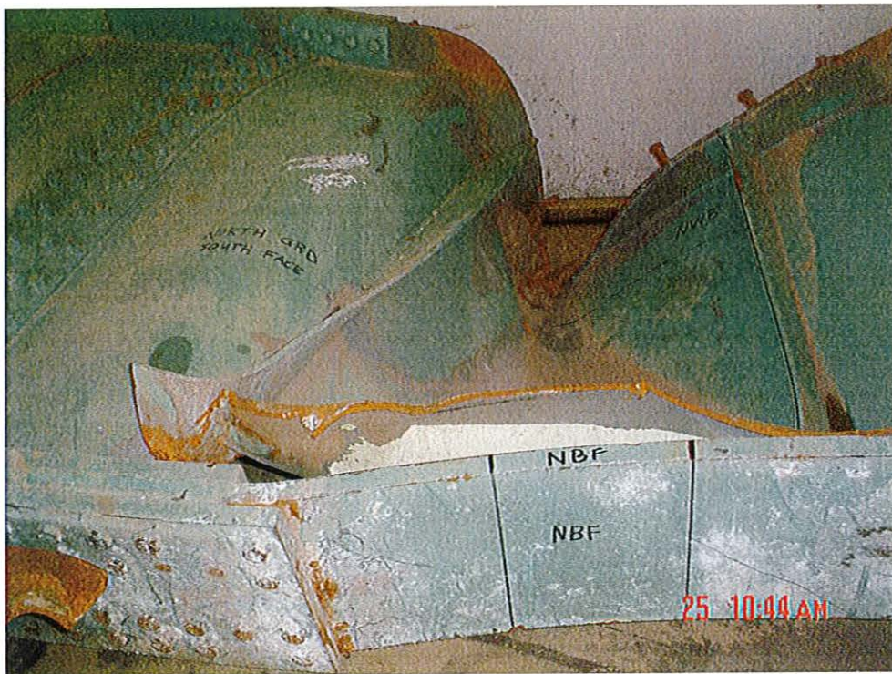
FIGURE 29 (North girder bottom flange)
