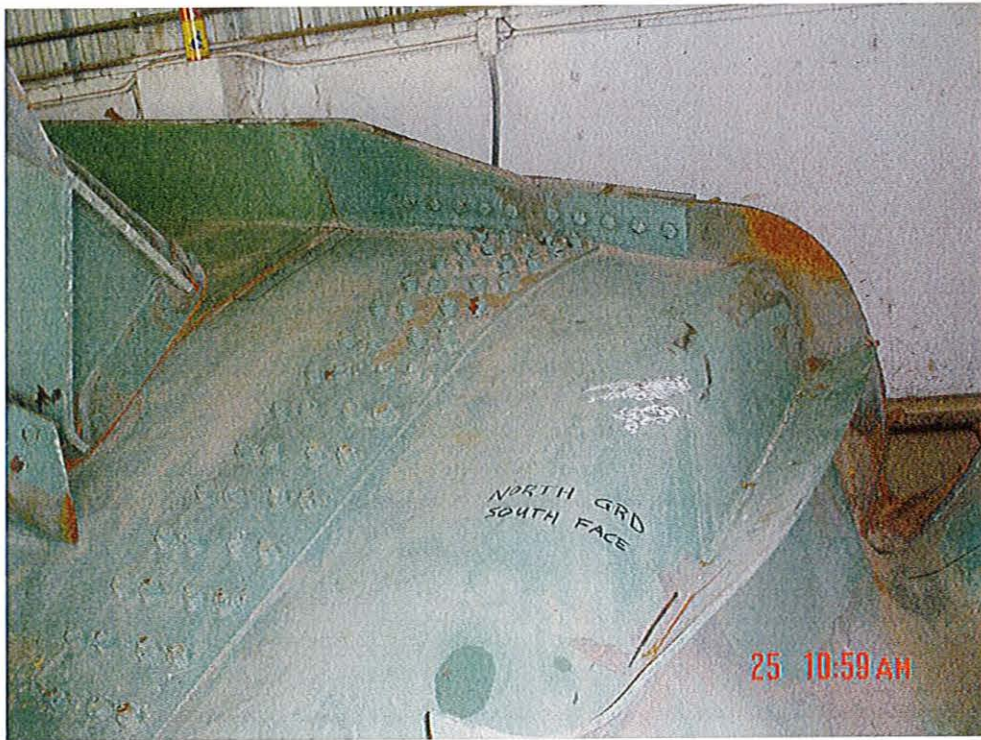
FIGURE 33 (North girder south face bottom flange)
