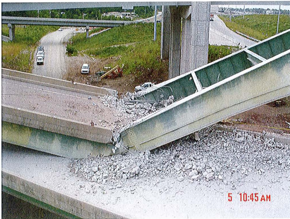
FIGURE 16 (Looking south, collapsed bridge girder span 2-3 fell on lower bridge into V-shape)
