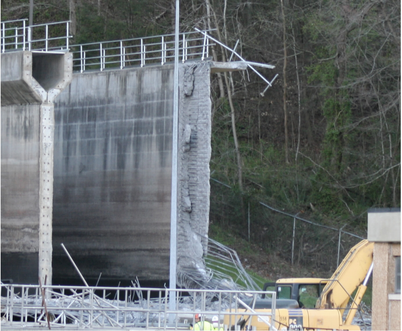
Fig. 6 Dowel Bars at the Corner Joint between the East Wall and North Wall (# 9 rebar @ 6" o.c., each face)
