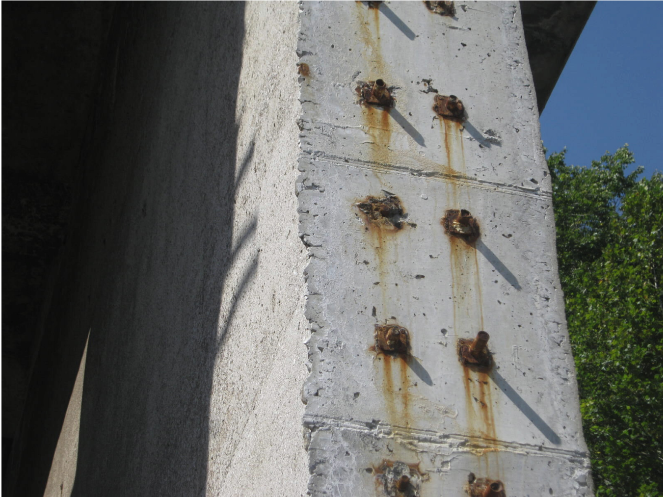
Fig. 2 Cold Joint between a Baffle Wall and the East Wall
