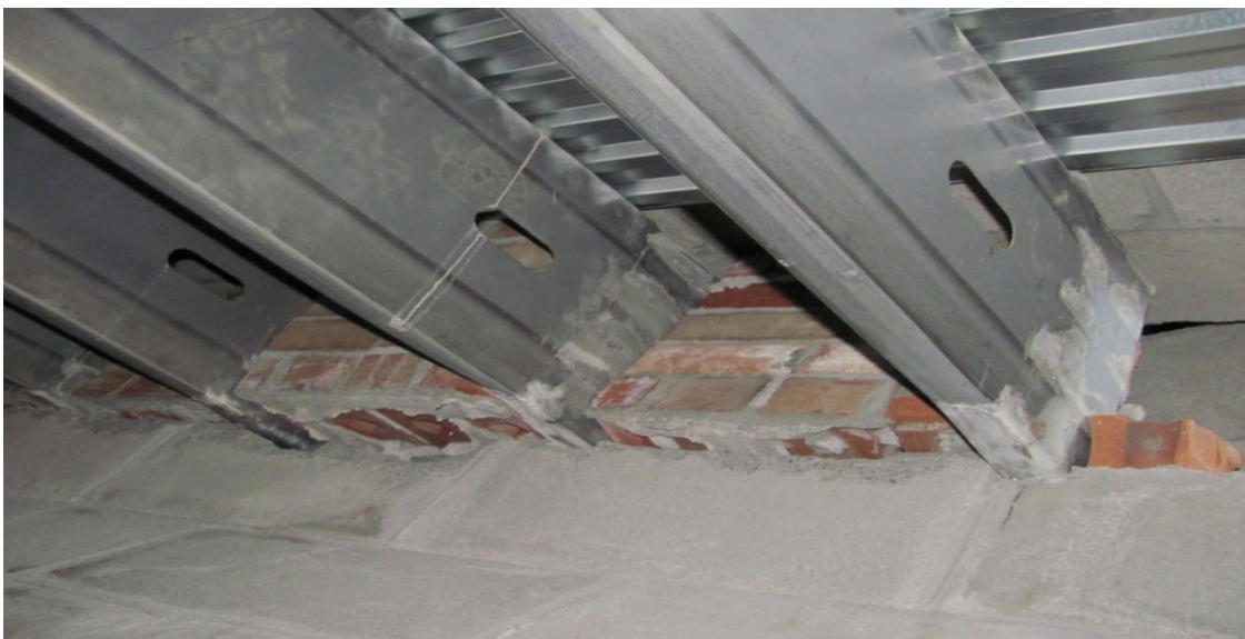
Fig. 7 C-joists blocked in by brick masonry.
