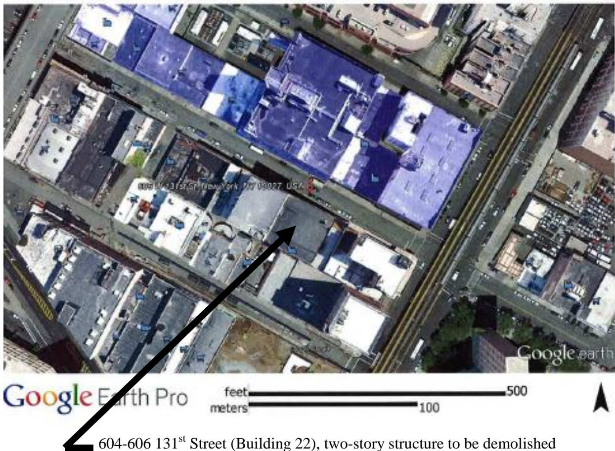
Figure 1 Aerial View of the Building
