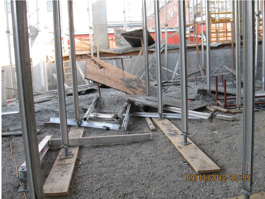
Figure 11. Another view of the base support of post shores.
