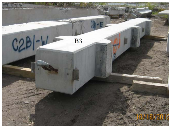
Fig. 41 – Column B3 upper segment in the yard
