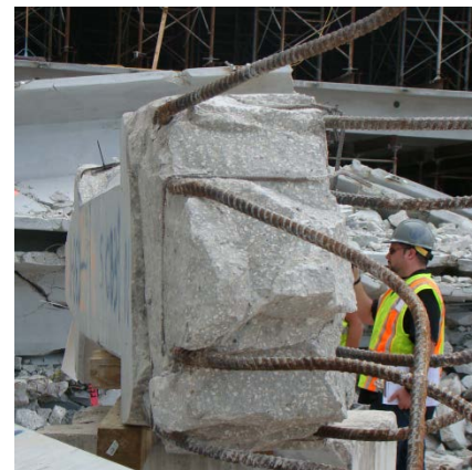
Fig. 44 – Column B3 lower segment
