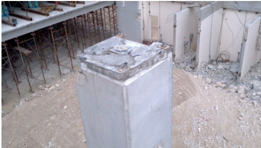
Fig. 56 – Grout at splice of B4 column
