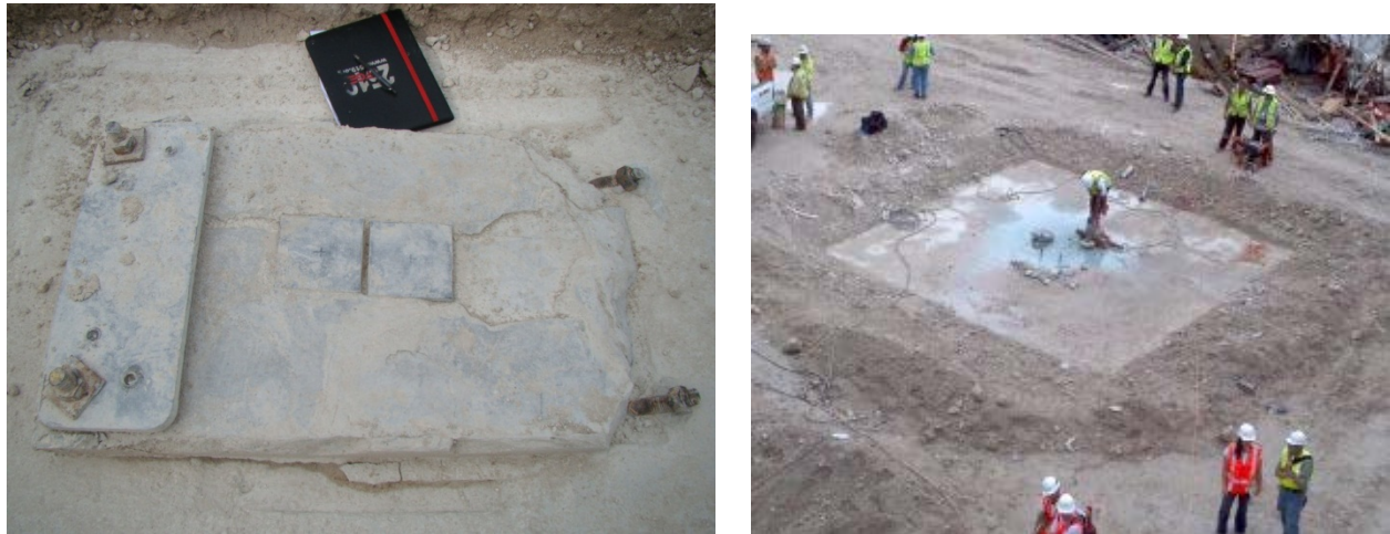
Fig. 35 – Base of column B2 after clean-up
