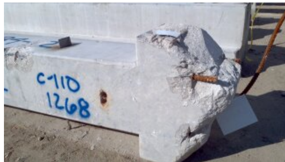
Fig. 53 – Column B4 upper segment above splice after demolition
