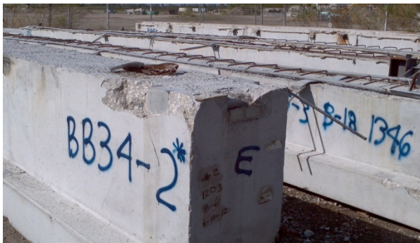
Fig. 68 – IT beam between B3 and B4 2 nd level in the yard
