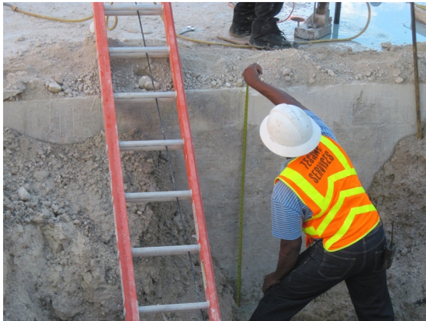
Fig. 72 – Exposed foundation for column B3
