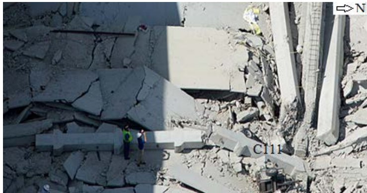
Fig. 42 – Column B3 lower segment fell towards south
