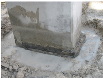
Fig. 58 – Base of column B4
