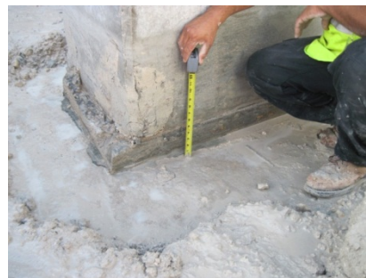
Fig. 59 – Grout at base of Column B4
