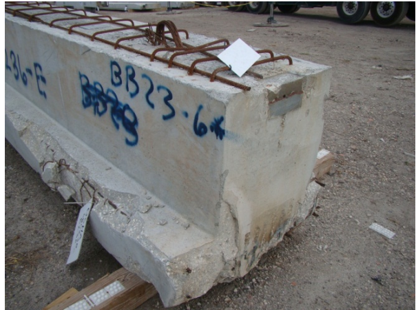
Fig. 67 – IT beam between B2 and B3 6 th level in the yard
