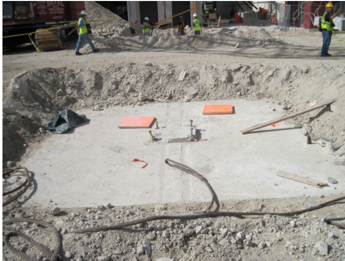
Fig. 60 – Footing for column A2
