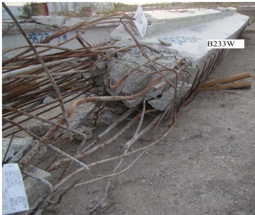
Fig. 64 – IT beam between B2 and B3 3 rd level in the yard
