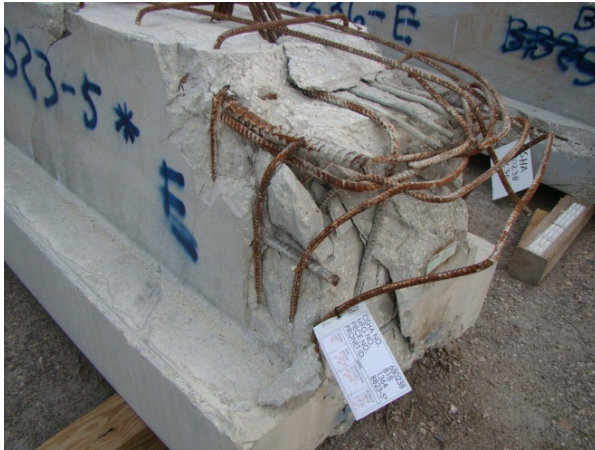
Fig. 66 – IT beam between B2 and B3 5 th level in the yard
