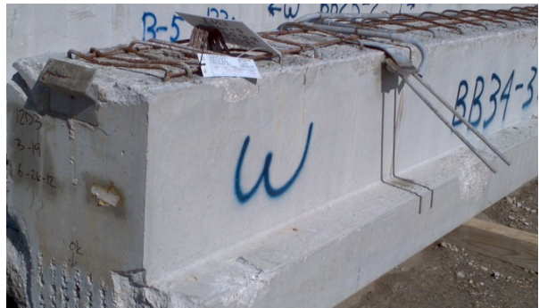
Fig. 69 – IT beam between B3 and B4 3 rd level in the yard
