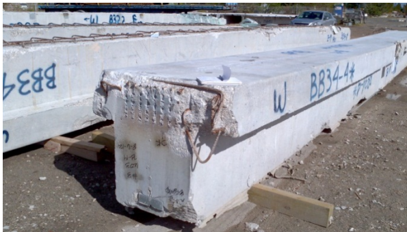
Fig. 70 – IT beam between B3 and B4 4 th level in the yard
