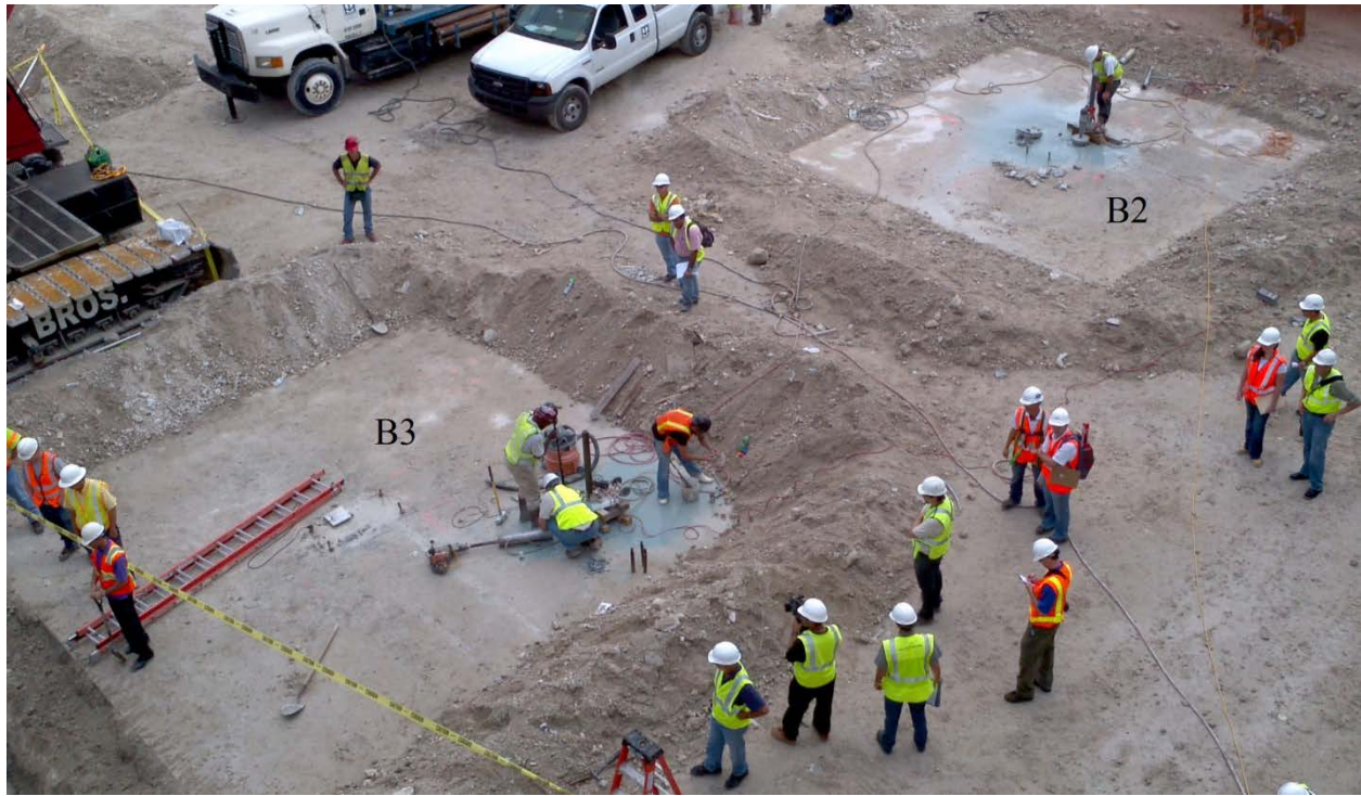
Fig. 34 – Foundation of column B2 and B3 after clean-up
