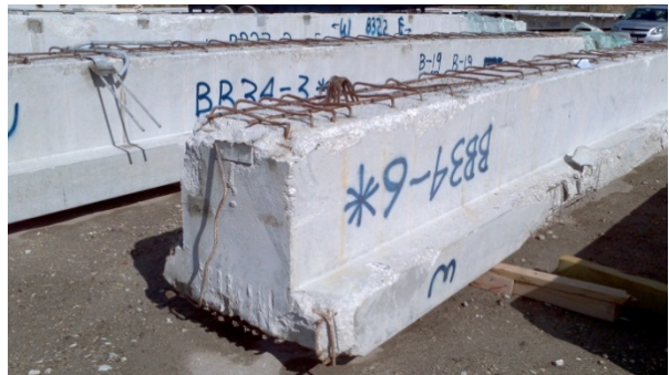
Fig. 71 – IT beam between B3 and B4 6 th level in the yard
