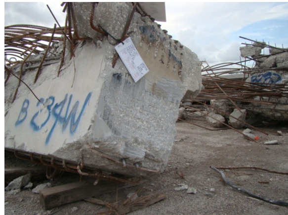
Fig. 65 – IT beam between B2 and B3 4 th level in the yard
