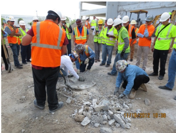
Fig. 46 – Base of B3 cleanup
