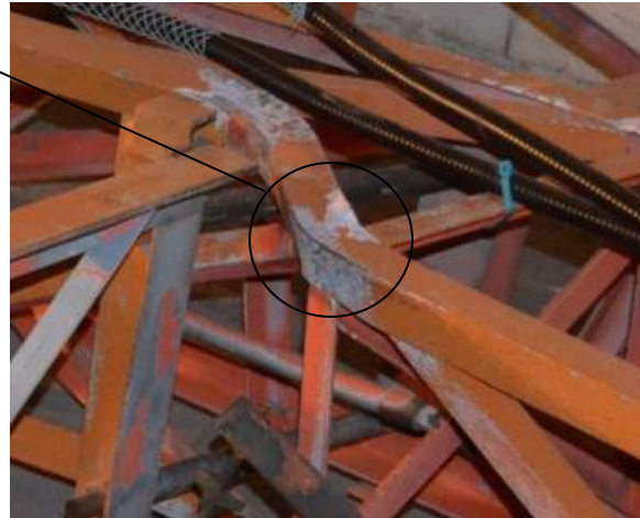
Figure 38 - Top block rigging location
