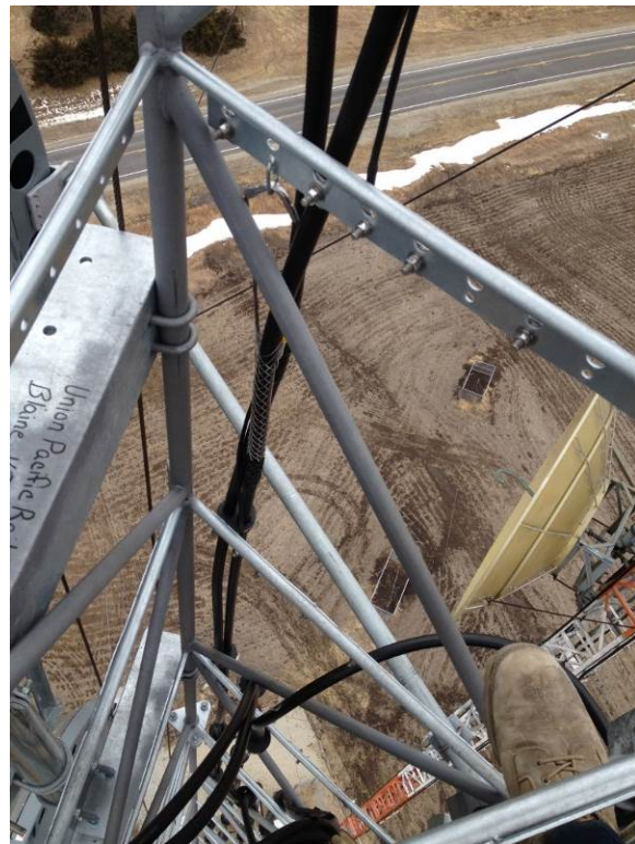
Figure 13 –Photo taken before collapse
