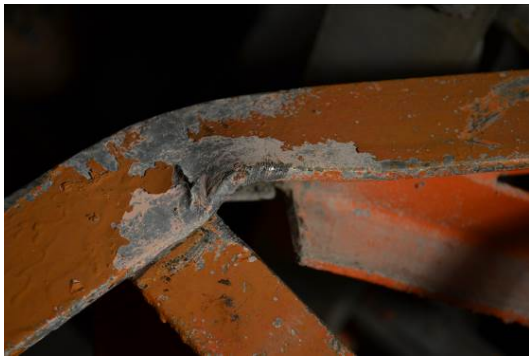
Figure 53 – Cuts and bruises from abrasion of wire rope
