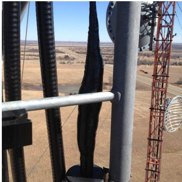
Figure 12 – Photo taken before collapse
