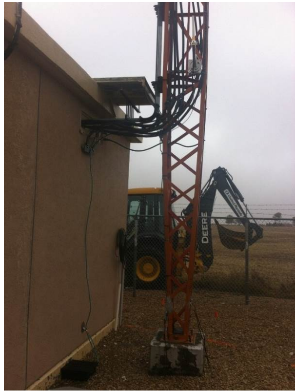
Figure 5 – Existing Tower – photo before collapse
