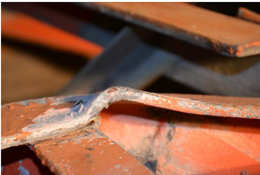
Figure 55 – cuts and bruises from abrasion of wire rope
