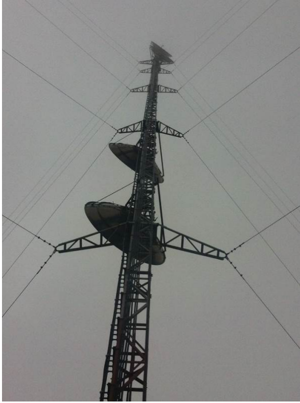
Figure 4 – Existing Tower – photo before collapse
