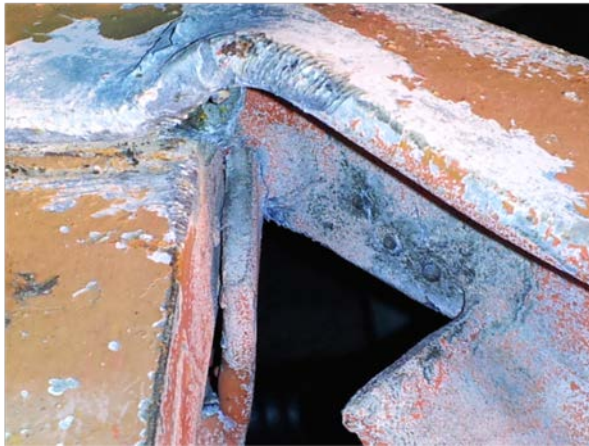
Figure 39 - Top block rigging location
