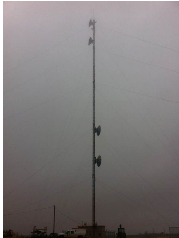
Figure 3 – Existing Tower – photo before collapse
