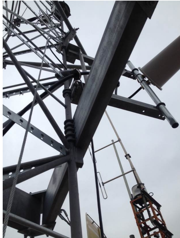
Figure 11 –Photo taken before collapse
