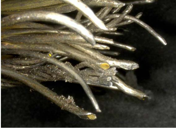
Figure 45 - Paint on fractured wire rope ends
