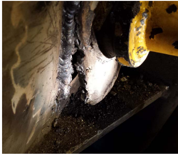
Fig. 10 – Failed weld showing lack of fusion
