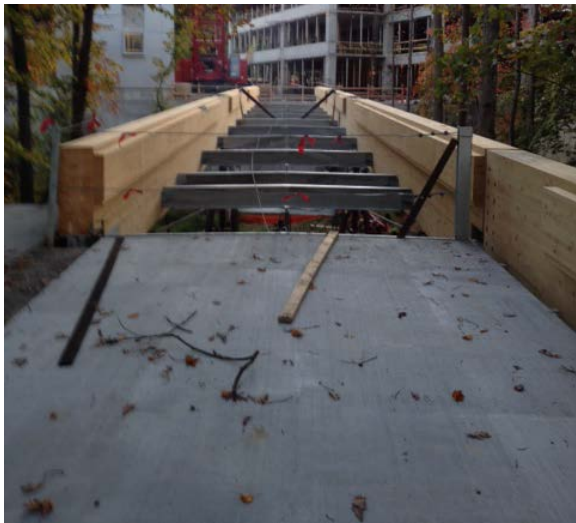
Fig. 50 – Framing for the deck
