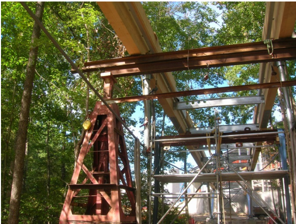
Fig. 46 – Temporary shoring tower supporting the trusses
