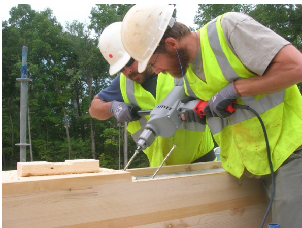
Fig. 52 – Screws being driven for splice flange plates
