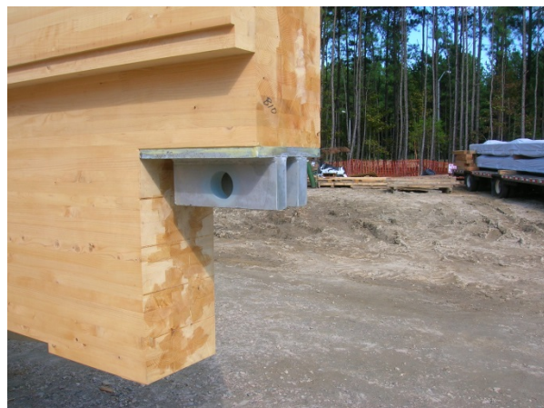
Fig. 53 – Sliding joint plates embedded in glulam girders
