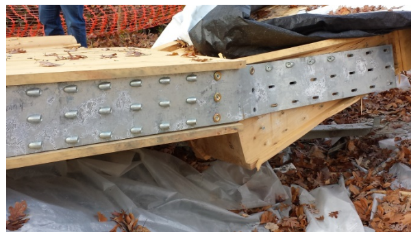
Fig. 30 – View of the top splice plates
