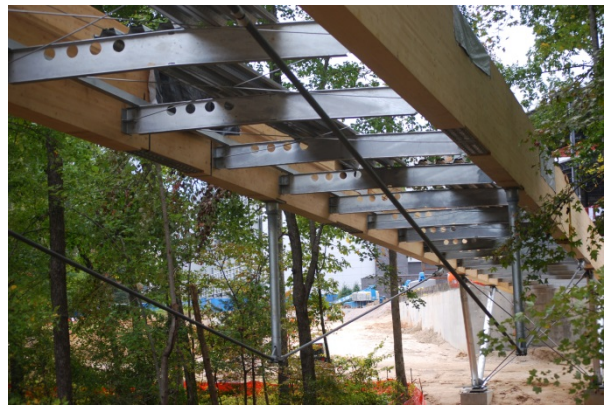
Fig. 47 – King post and the cables
