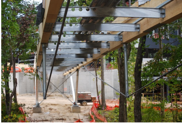
Fig. 48 – Cables being positioned
