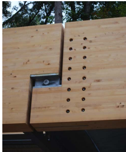
Fig. 51 – Sliding joint between glulam girders
