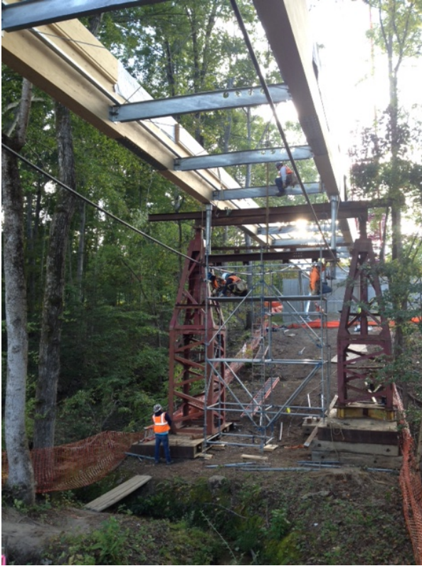
Fig. 44 – Temporary shoring tower supporting the trusses
