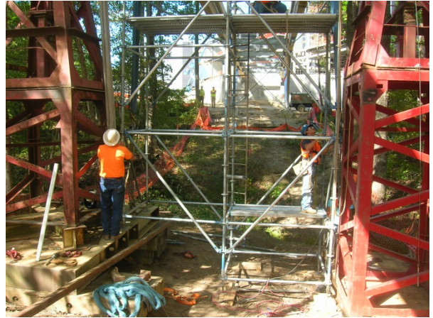
Fig. 45 – Temporary shoring tower
