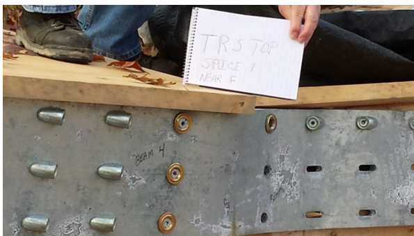
Fig. 29 – View of the top splice plates
