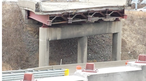
Figure 14 – West pier (pier #1) and abutment #1
