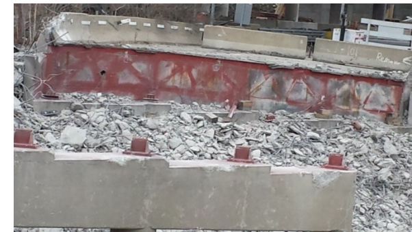
Figure 18 – Another view of Pier #2 and abutment #2
