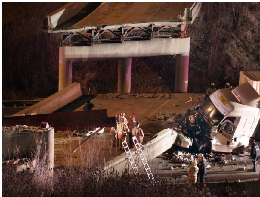
Figure 10 – I-75S after the incident (taken from the web)
