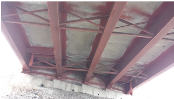
Figure 15 – West span girders and cross frames
