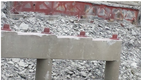
Figure 17 – Pier #2 and abutment #2
