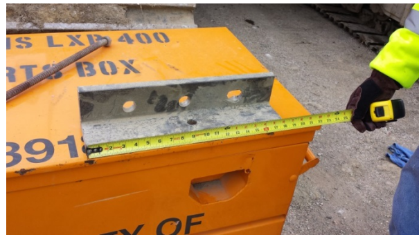
Figure 22 – Another view of 4x4x3/4" angle used at abutment #2
