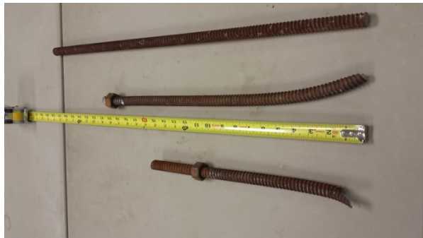
Figure 23 – 3/4" coil rod that was used at abutment #2 to hold down the girder
