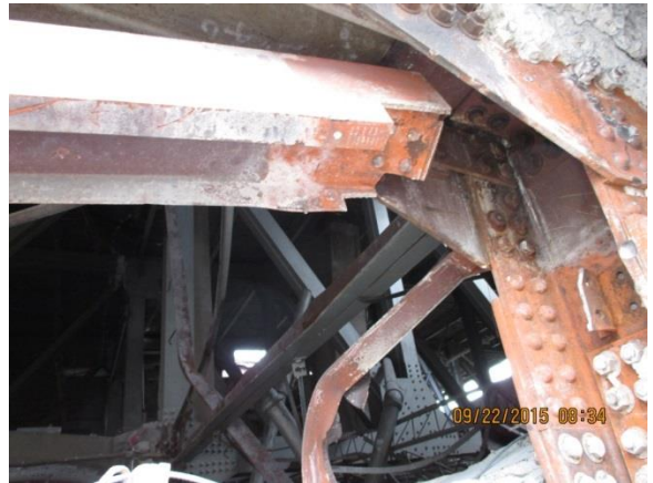
Partial north view FIGURE 16
