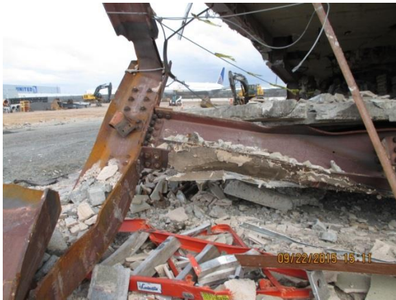
Partial west view at column line A14 FIGURE 9
