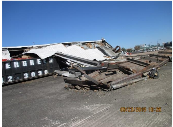
Partial east view at column line H14 FIGURE 20
