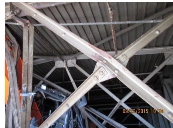
Partial east view for cantilever truss FIGURE 24
