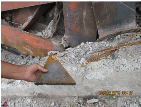
Partial north view FIGURE 17
