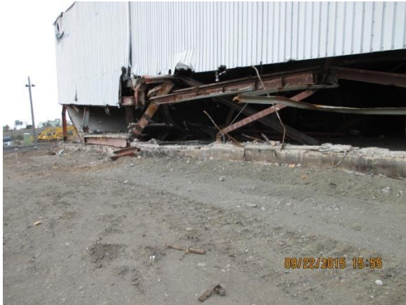
Partial south view from column line A1 FIGURE 25
