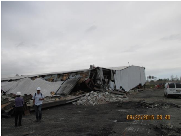
Partial north-east view from column line H14 FIGURE 19
