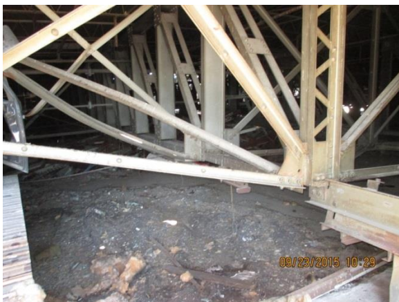
Partial east view for cantilever truss FIGURE 23
