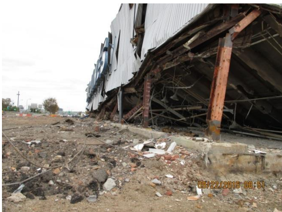
Partial west view from column line A1 FIGURE 29
