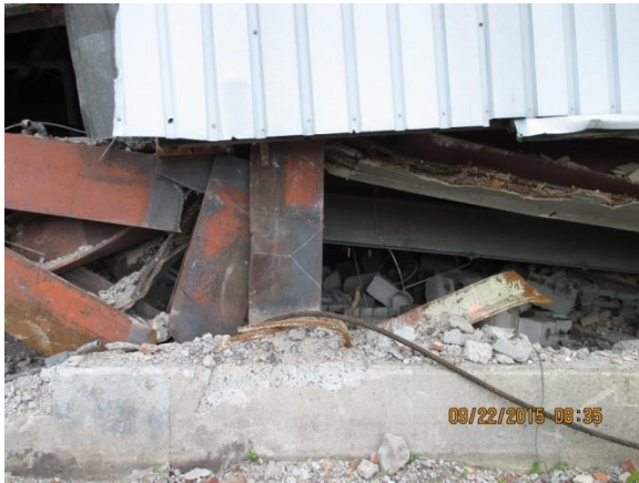
Partial north view FIGURE 15
