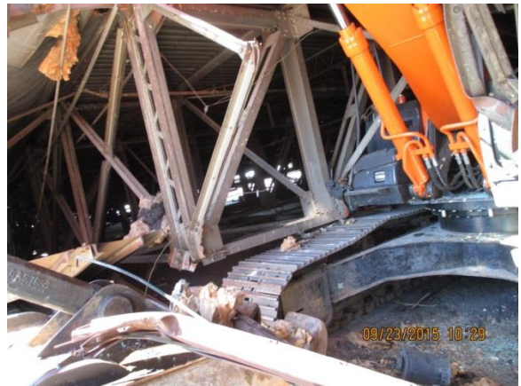
Partial east view where excavator trapped FIGURE 22
