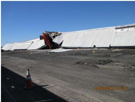
Partial east view where roof held by excavator FIGURE 21
