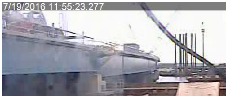
(Pile driving in progress)
