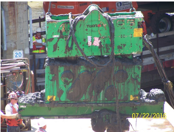
Fig. 26 - Vibratory Hammer recovered from water
