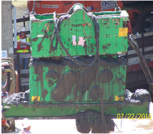
J&M vibratory hammer 66
