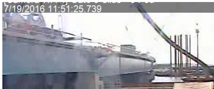
(Pile driving is already in progress.)
