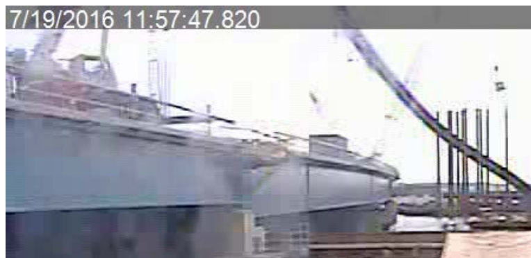
(Vibratory hammer released and swinging towards the boom at 11:57:47 a.m.)
