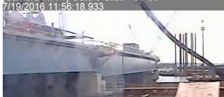
(Shows Pile extraction.)
