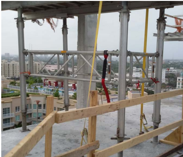
Fig. 9 – Formwork tables installed by table-setting crew. Fig. 10 – Formwork table installed by table-setting crew.
