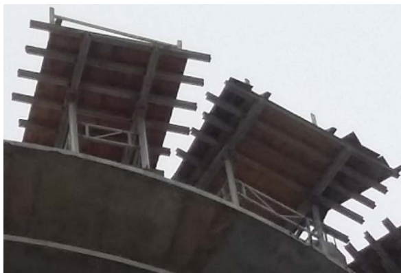
Fig. 7 – Formwork tables installed by table-setting crew. Fig. 8 – Formwork table installed by table-setting crew.
