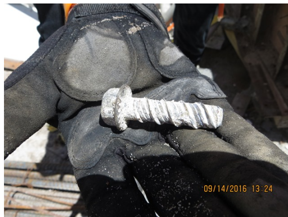
Fig. 17 – Wedge-Bolt Screw Anchor found in debris.
