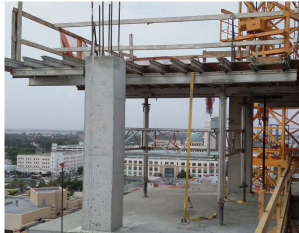
Fig. 9 – Formwork tables installed by table-setting crew. Fig. 10 – Formwork table installed by table-setting crew.
