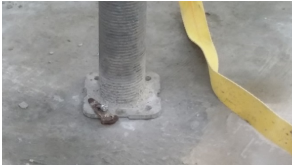
Fig. 20 – EZ post anchoring.
