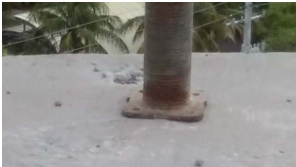
Fig. 22 – EZ post anchoring. (no screws)
