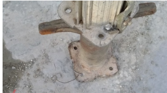
Fig. 21 – EZ post anchoring with nails.
