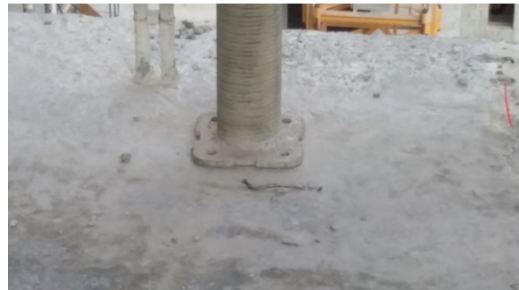
Fig. 23 - EZ post anchoring. (see the nail)
