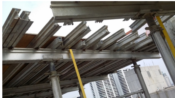
Fig. 7 – Formwork tables installed by table-setting crew. Fig. 8 – Formwork table installed by table-setting crew.
