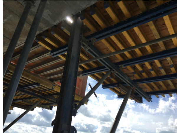
Fig. 7 – Scaffold in stationary position
