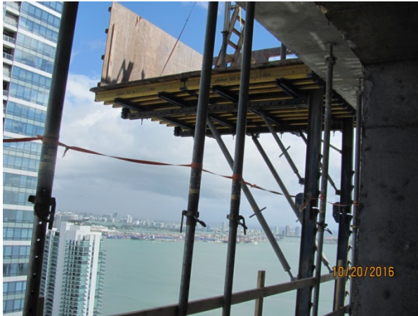
Fig. 6 – Scaffold in stationary position
