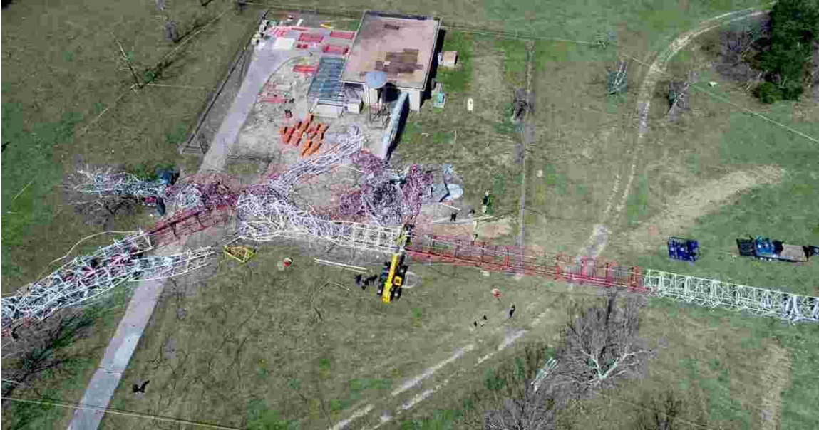
Figure 5. Collapsed Communication Tower (Google Image Search)
