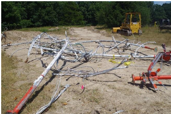
Figure 7. Recovered Section of the Tower 90'-120'
