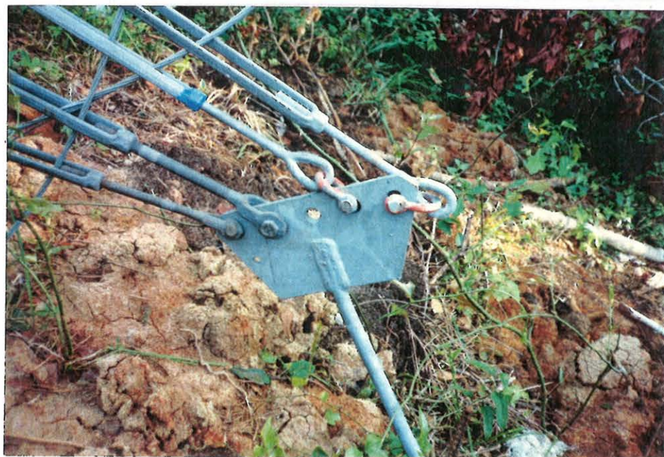
Three outer anchors-showing exposed steel rods
