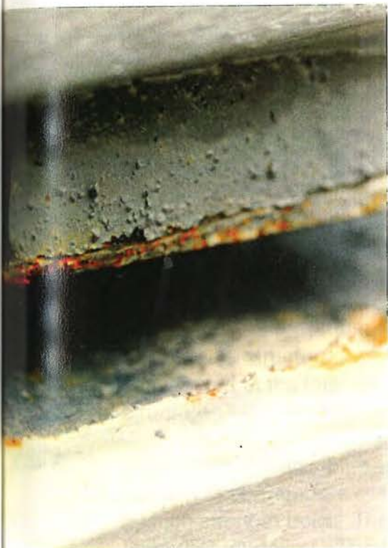
Fractured Weld in a Spacer Between a Joist Chord
