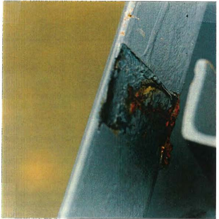
Fractured Welds in Diagonal Member Spacers Between Top and Bottom Chords
