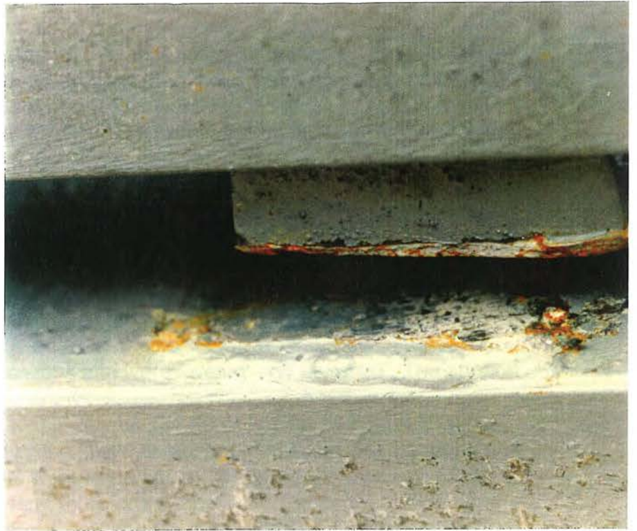
Fractured Weld in a Spacer Between a Joist Chord
