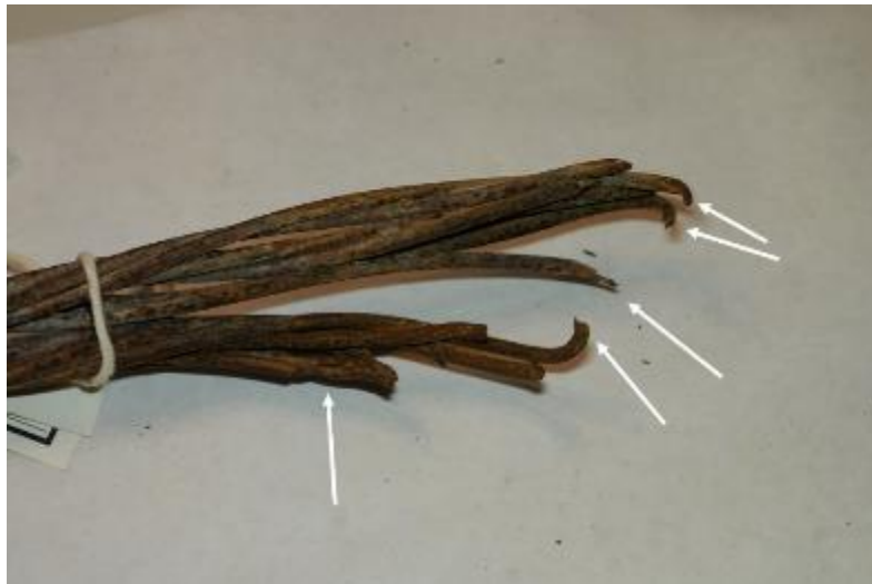
Figure 7: Failed end of Sample 1. The white arrows point to wire ends that failed in corrosion-assisted brittle failure. Also note several of the wires were bent around a small radius, which contributed to the failure.
