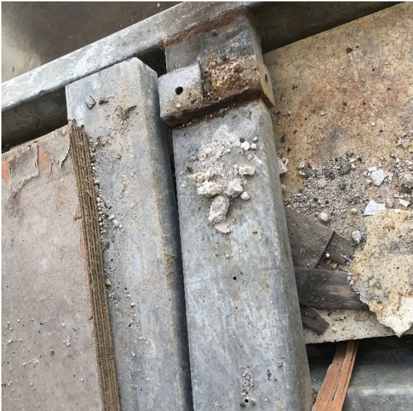
Figure 20 – Connection to the hotel (east support)
