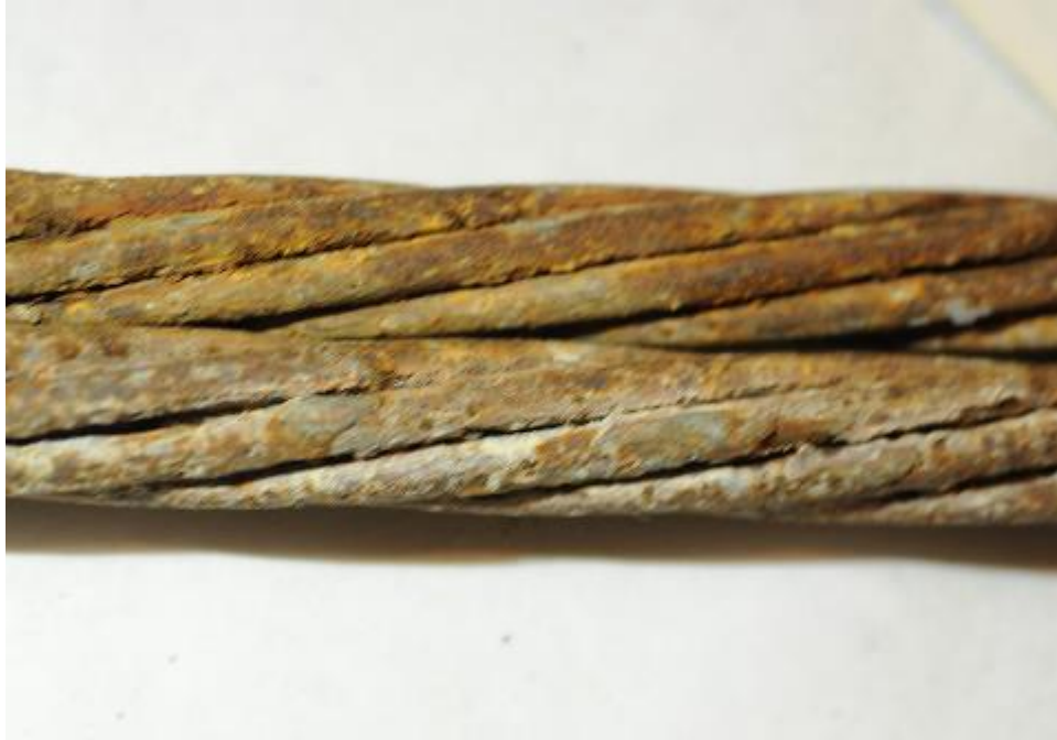
Figure 10: Example of the corrosion on the wire rope. Sample 4
