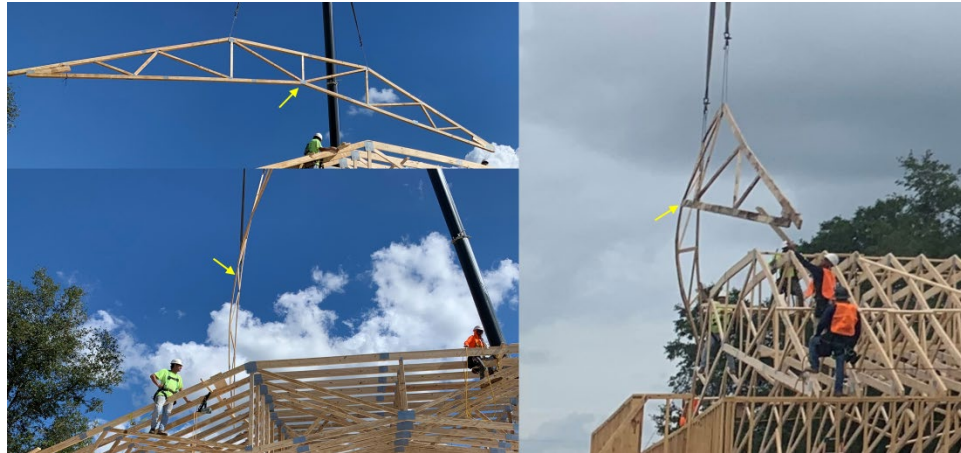
Figure 15 – Truss hoisting (Photo by WW Build)
