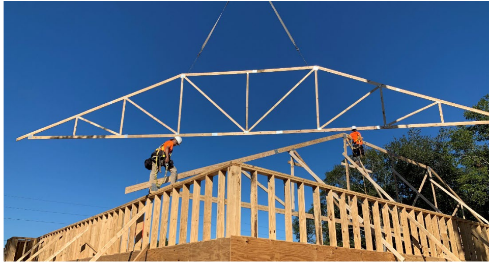
Figure 7 – Truss erection – looking northwest (Courtesy of WW Build)
