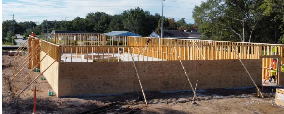
Figure 3 – Bearing walls – looking west (Courtesy of WW Build)
