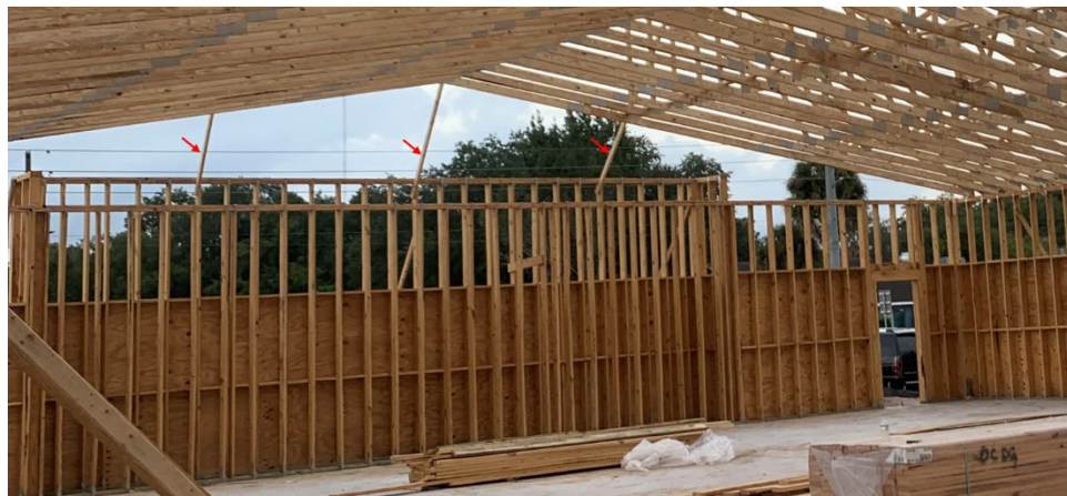
Figure 9 – Truss diagonal end braces at the west side – looking west (Photo by WW Build)
