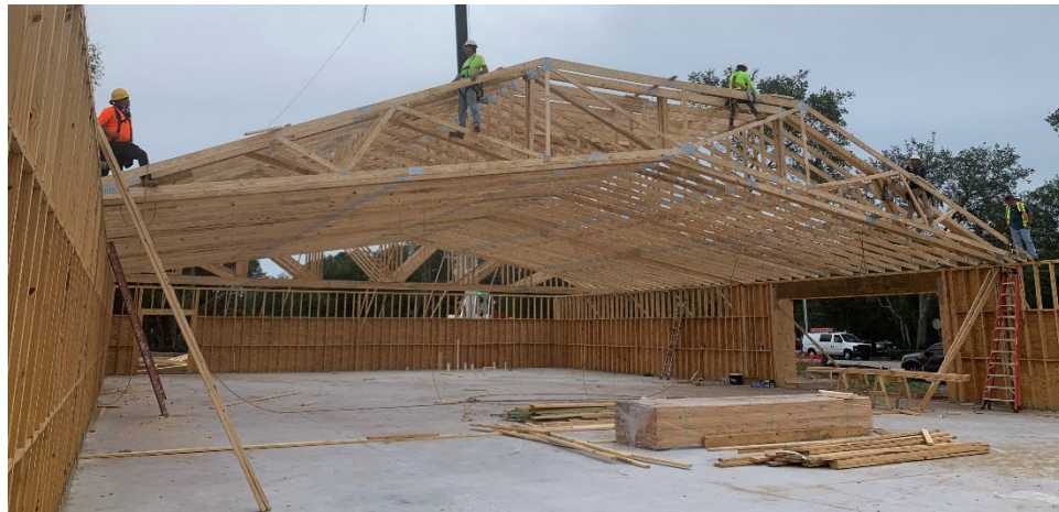
Figure 4 – Bearing walls and trusses – looking east (Courtesy of WW Build)
