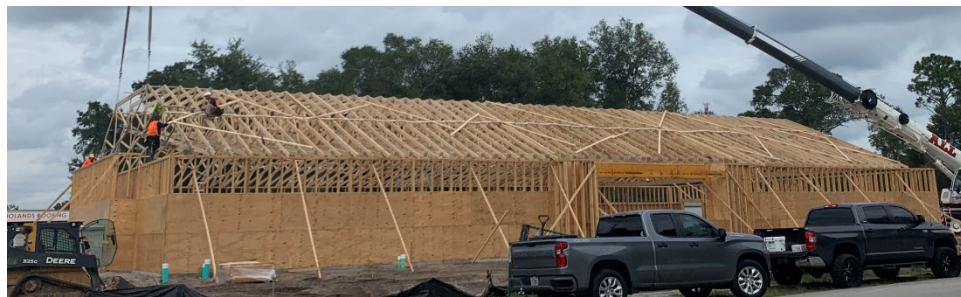
Figure 5 – Bearing walls and trusses – looking north (Courtesy of WW Build)
