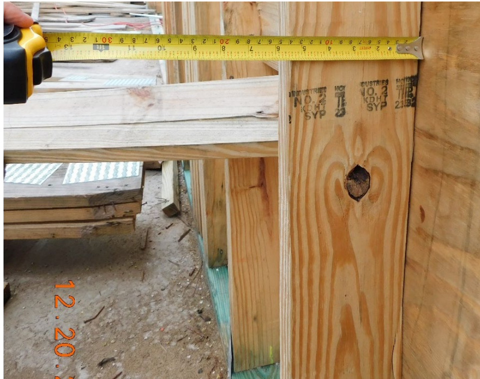
Figure 21 – Bearing wall frame – studs
