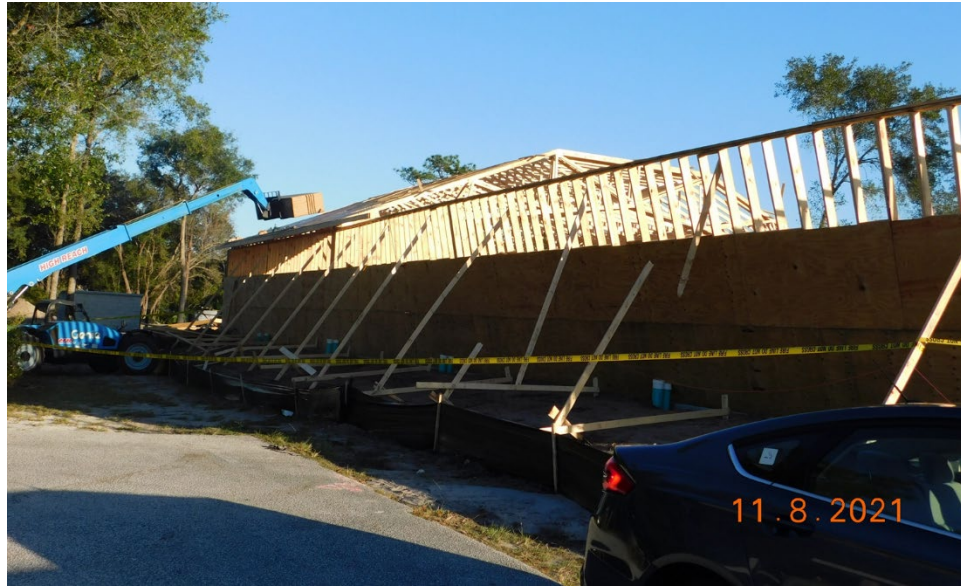
Figure 10 – Wall diagonal braces at the north side – looking southeast
