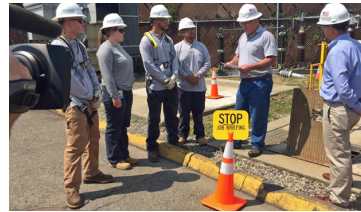
Eversource management (at right) waits to be fully briefed and signed into the work area, while the crew leader finishes a pre-job brief with other workers.
