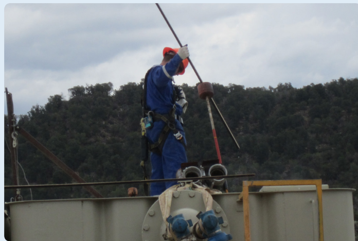
A worker manually gauges a flowback tank. The thief hatch is directly in front of his feet, and the gas and vapor released is invisible. Image: Max Kiefer, NIOSH.
